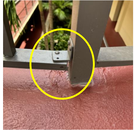
Photo # 13 Missing Fasteners on Railing Bracket
