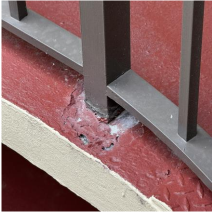
Photo # 11 Deteriorated Railing Post Pocket
