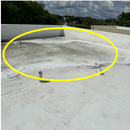
Photo # 15 Signs of Water Ponding
