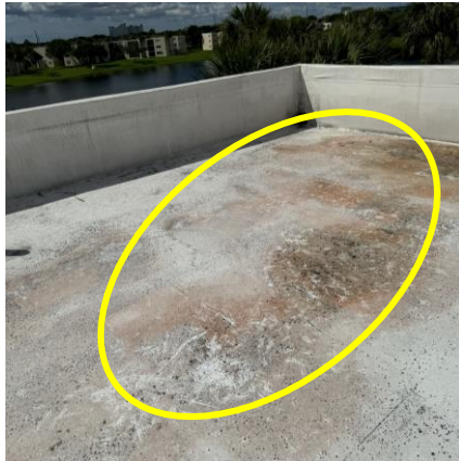
Photo # 16 Signs of Water Ponding
