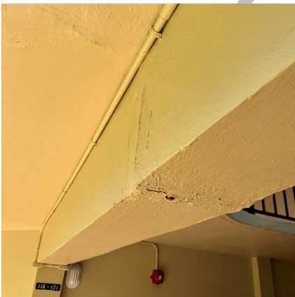
Photo # 7 Deteriorating Expansion Joint
