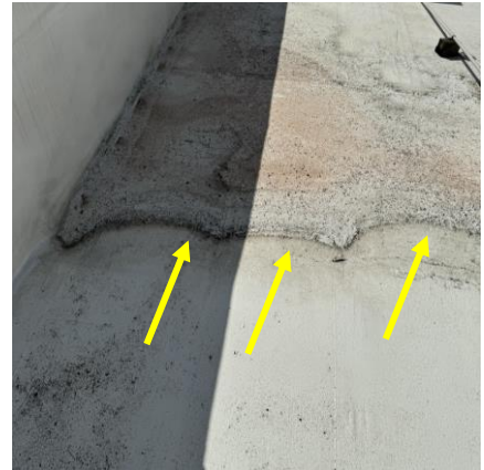
Photo # 17 Improper Waterproofing Application
