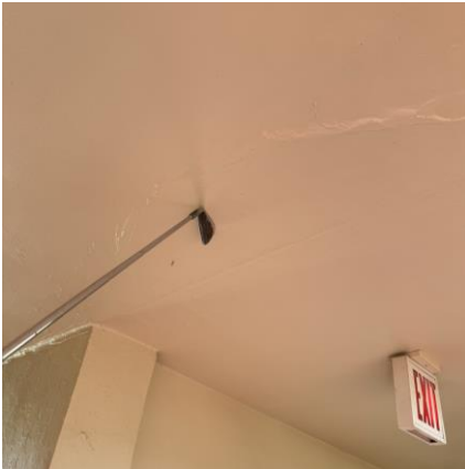
Photo # 1 Spalled Concrete
