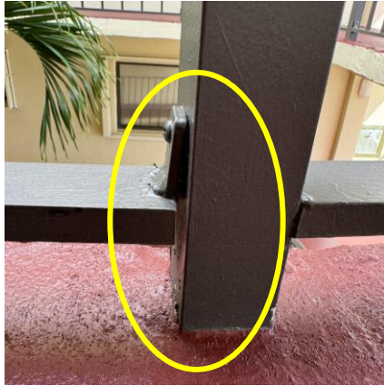
Photo # 12 Deteriorated Railing Bracket
