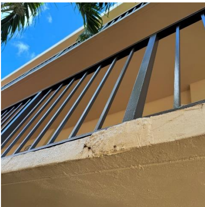
Photo # 4 Spalled Stucco/Concrete
