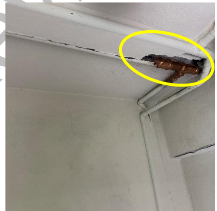
Photo # 6 Improper Slab Cut for Pipe Installation.
