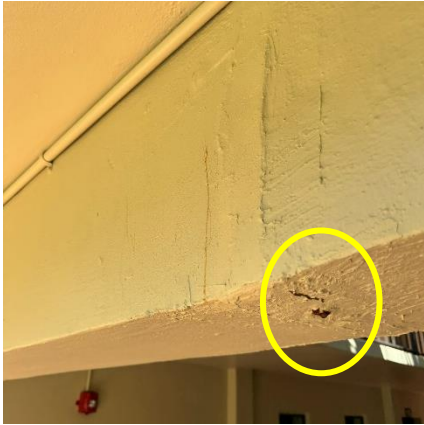
Photo # 9 Corroded Rebar Pop Out
